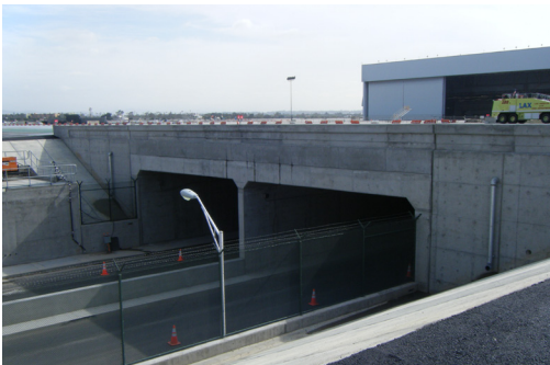
LAX - NEW TAXIWAY BRIDGE
