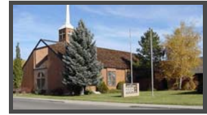
Bethlehem Lutheran Church and School -- energy-efficient electrical systems
